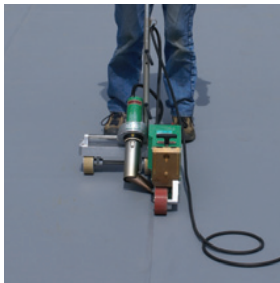
Using a hot-air welding machine
