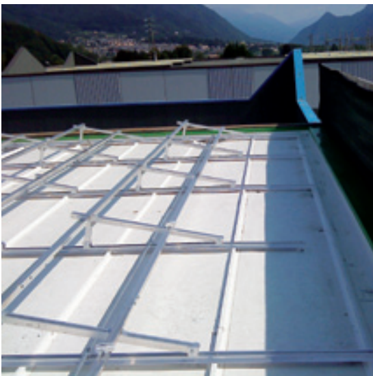
RENOLIT ALKORSOLAR – your solar panels are fixed without any perforation of the waterproofing membrane.
